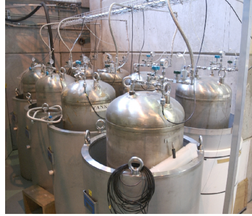
Figure 3.48: Gas xenon storage tank.
