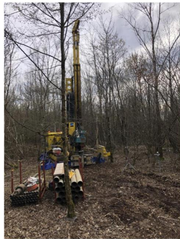
➤ Drilling machine in place
