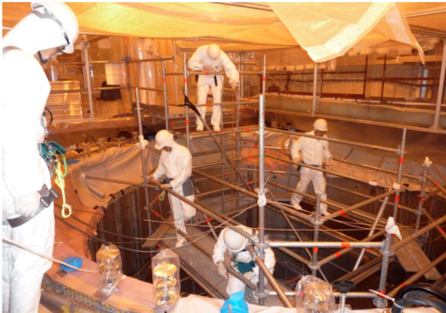
DC-Japan PMT 設置作業 2009.5 @ Chooz suekane@ICEPP
